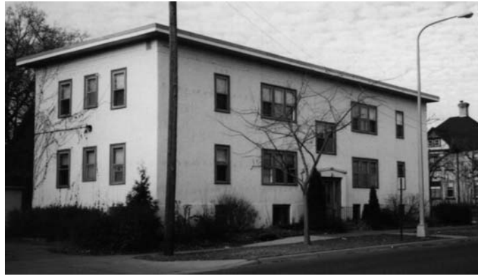
333 Fourth Avenue South
