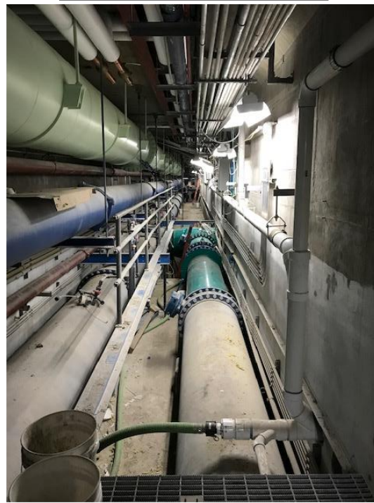
In Progress of Removal
